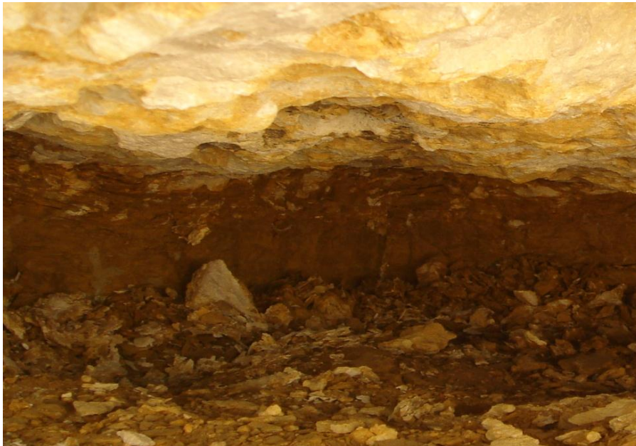
Cavity encountered under bridge abutment – not shown on BH log, no GI supervision
